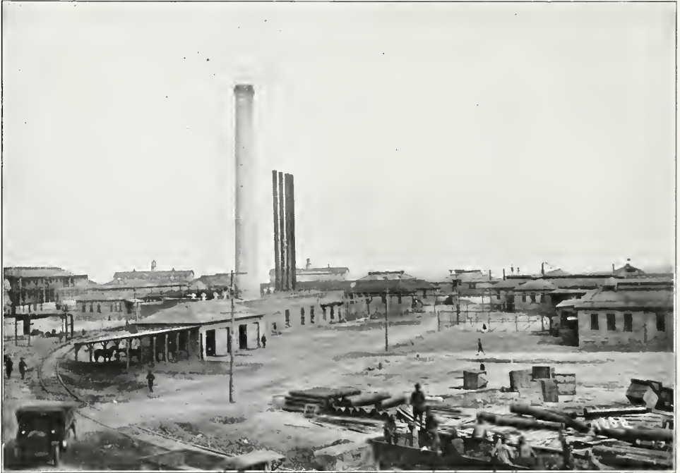
FIG. 160.—General view of Embarkation Hospital, Newport News, Va., showing central heating plant.
